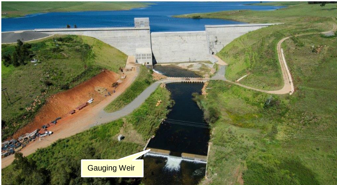
Figure 22: Example of a gauging weir downstream of Spring Grove Dam
