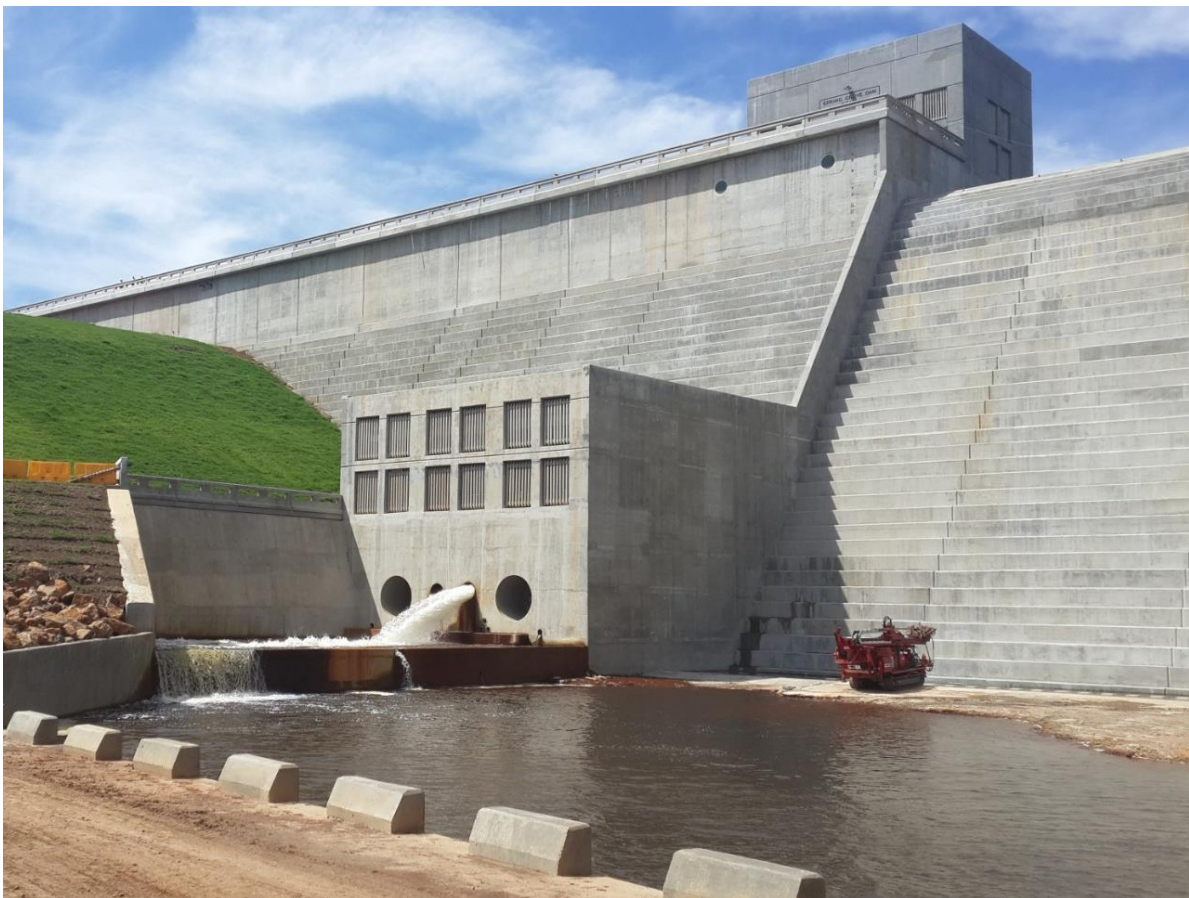
Figure 29: Example of controlled release from outlet works at an RCC dam type (Spring Grove Dam)
