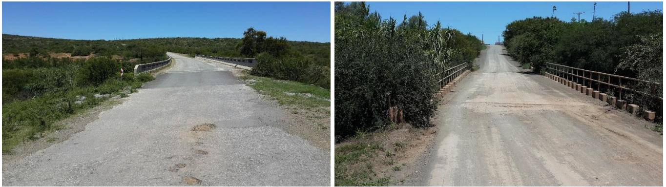
Figure 16: Photographs of existing R344 (bridge structures shown)
