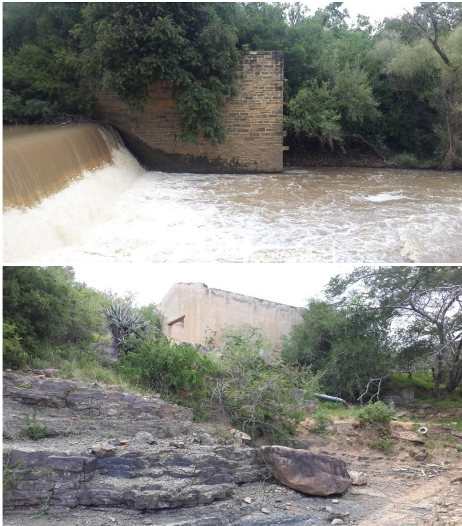
Figure 77: Stone weir (top) and old pump house (bottom)
