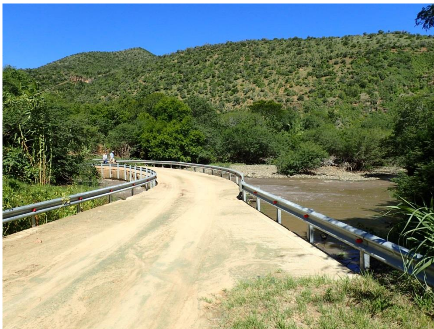
Figure 25: Photograph of existing drift along DR 02491
